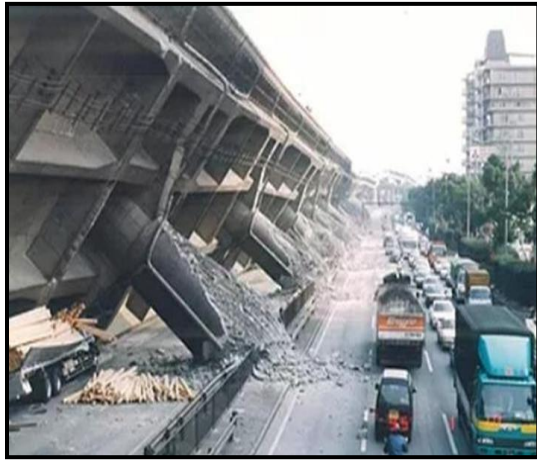
Fig (44): Bridge collapse due to earthquake
