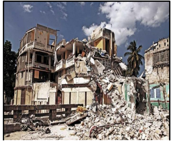
Fig (45): Building Collapse due to earthquake
